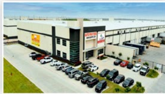
Safe Pro House: Village Pogaon, Taluka Bhiwandi, District, Thane - 7421 302
